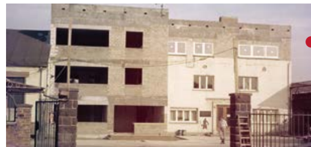
Expansion of the headquarter in Andernach
